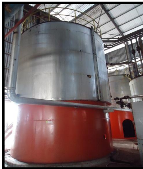
Gambar 1 Continuous Settling Tank (CST)
